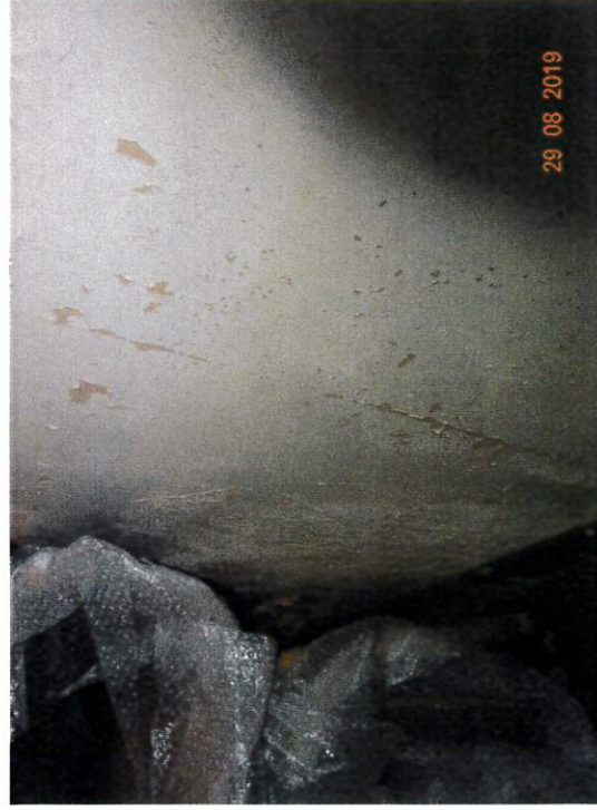
Damp wall area-rear ground floor store
