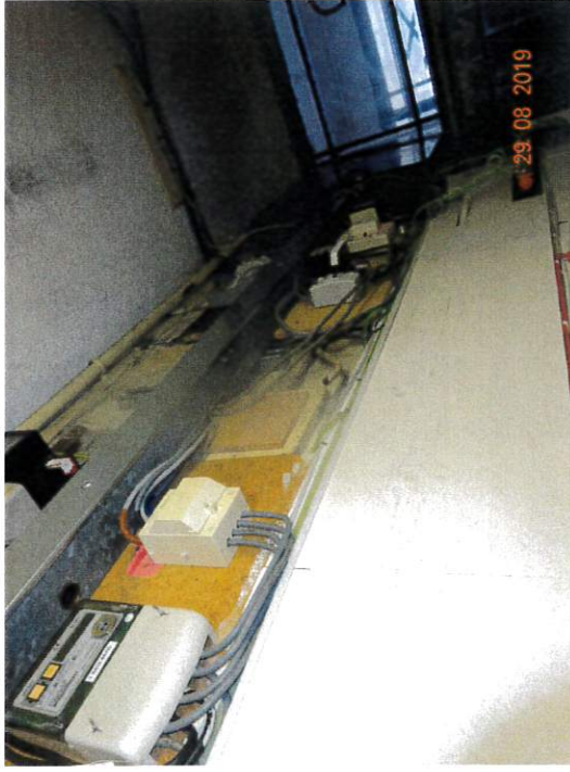
Exposed Wiring-Rear Ground Floor Hallway
