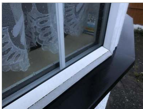
Photo - 25 Upvc double glazed windows appear functional but are externally beaded which may be a security concern.
