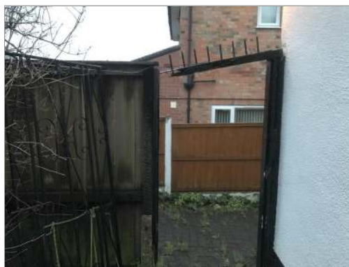
Photo - 40 Remove nails to broken side gate frame to avoid various liability claims.
