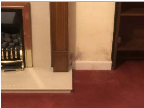
Photo - 93 Low level blown plaster noted to lounge chimney breast.
