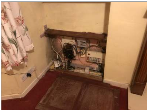
Photo - 109 Upgrade dated fusebox to lounge meter cupboard to split load rcd protected consumer unit.
