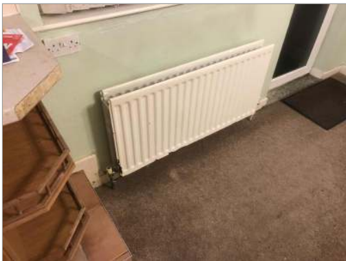
Photo - 113 Upgrade dated panel radiators to modern convector type.
