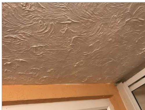
Photo - 67 Joint repairs required to artexed ensuite ceiling.
