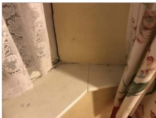
Photo - 76 More movement noted. Structural engineering consultation required.
