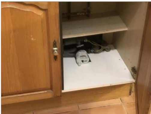
Photo - 112 Water meter and stop tap noted to base unit.
