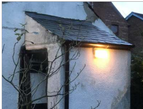
Photo - 11 Refix slipped slates to rear outhouse. Or renew.
