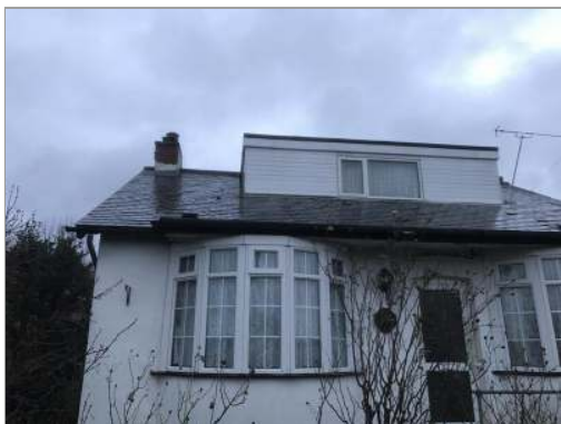
Photo - 4 Undulation noted to slated roof. Consider renewal for age related purposes.
