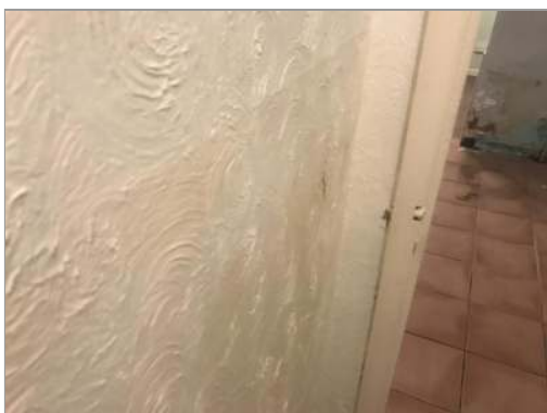
Photo - 69 Patch repairs required to artexed stud partition to bathroom and rear lobby. Test for asbestos before disturbing.
