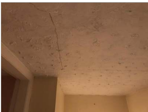
Photo - 66 Joint repairs required to artexed top floor bed 2 ceiling.
