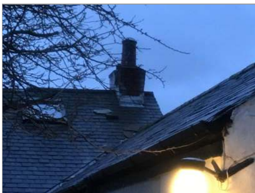
Photo - 3 Redress flashings, Repoint work brickwork.
