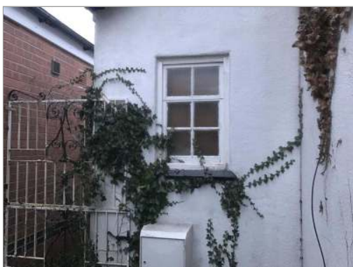
Photo - 24 Upgrade single glazed timber windows for thermal efficiency purposes.
