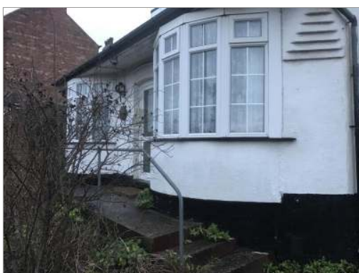
Photo - 16 Movement noted to front bay render.
