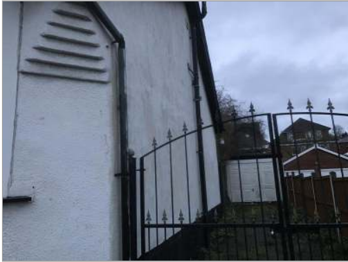
Photo - 18 Penetrative dampness noted to side elevation render.
