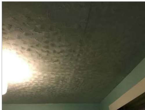
Photo - 63 Joint repairs required to rear bed 1 artexed ceiling.
