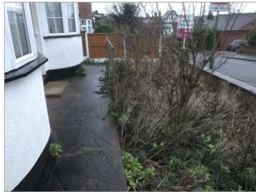
Photo - 49 Resin repairs required to cracked path to front.
