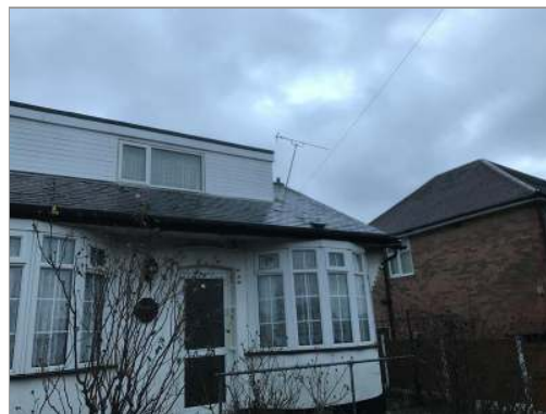
Photo - 5 Renew flashings around dormer.
