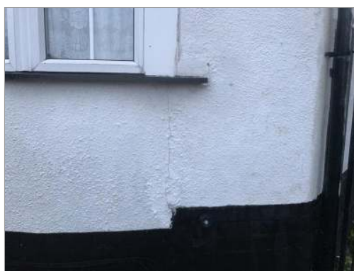
Photo - 17 Differential movement noted to front bay.
