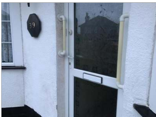
Photo - 31 Upvc front door noted. Ensure glazing is made shatterproof.
