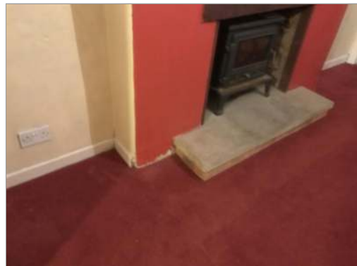
Photo - 94 Renew missing skirting to hearth.
