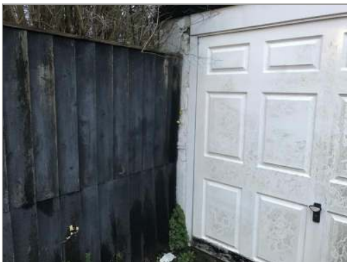
Photo - 128 Renew door which does not fully close at base. Incorrectly sized.
