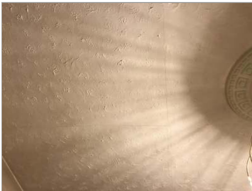
Photo - 62 Joint repairs required to artexed lounge ceiling.
