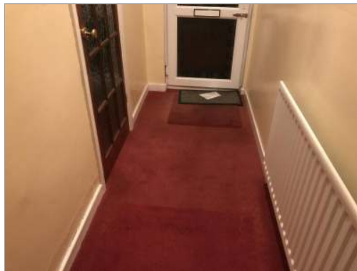
Photo - 88 Pack up sloping floor to landing.
