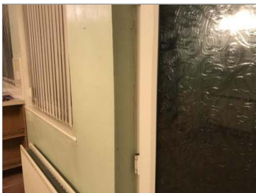
Photo - 73 Movement noted to rear door reveal.
