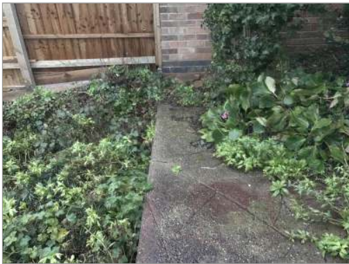
Photo - 48 Resin repairs required to cracked path.
