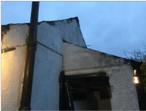
Photo - 28 Remove render and make good brickwork underneath or renew with insulated render.
