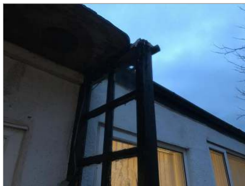
Photo - 34 Timber single glazed rear porch frame requires upgrading.
