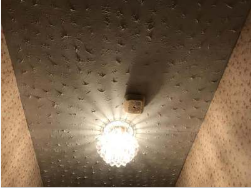
Photo - 108 Smoke detector noted to hallway.
