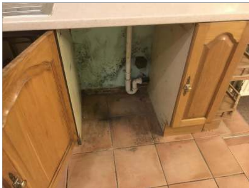
Photo - 71 Mould noted to kitchen wall.
