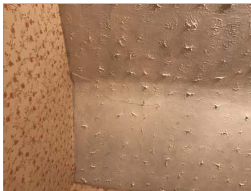
Photo - 65 Movement noted to landing staircase artexed ceiling.
