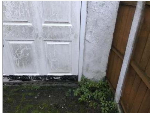
Photo - 127 Remove vegetation and low level rising dampness noted.
