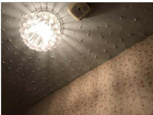
Photo - 64 Joint repairs required to artexed hallway ceiling.
