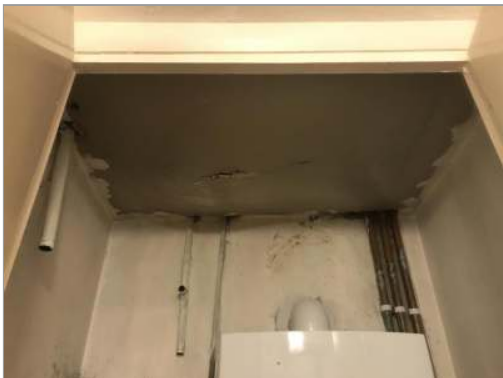
Photo - 96 Penetrative dampness noted to boiler cupboard from pitched roof above.
