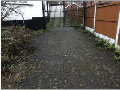
Photo - 52 Remove vegetation from front pavers and rebed.
