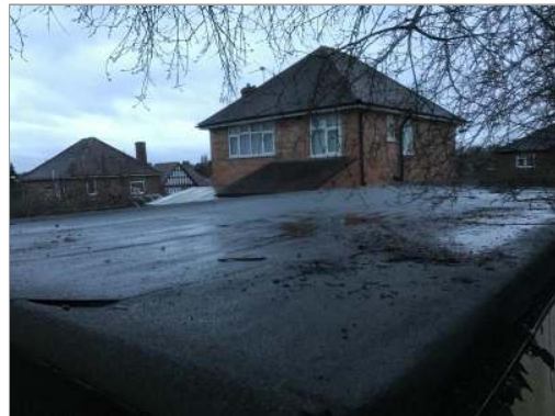
Photo - 117 Ponding noted to flat roof. Renew felt covering to roof and remake falls.
