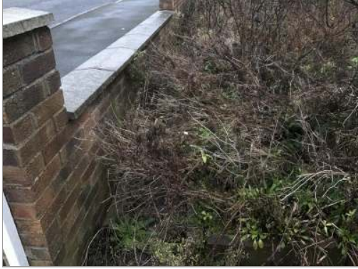
Photo - 50 Repoint copings and worn mortar to brickwork to front boundary wall.
