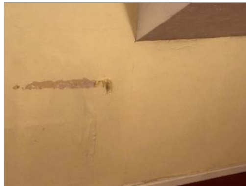
Photo - 84 Minor movement noted to rear wall to bed 2.
