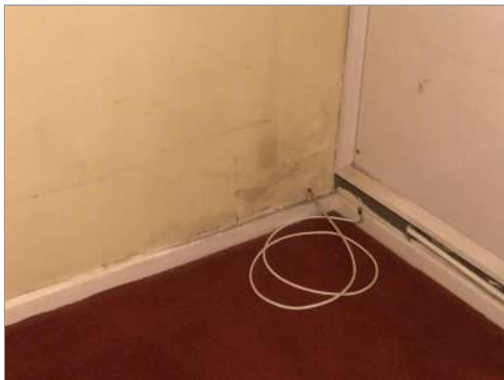
Photo - 83 Poorly plastered wall noted to bed 2.
