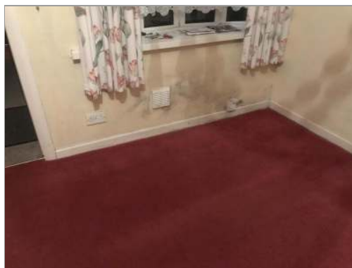
Photo - 74 Low level damp plaster and mould noted to dining room.
