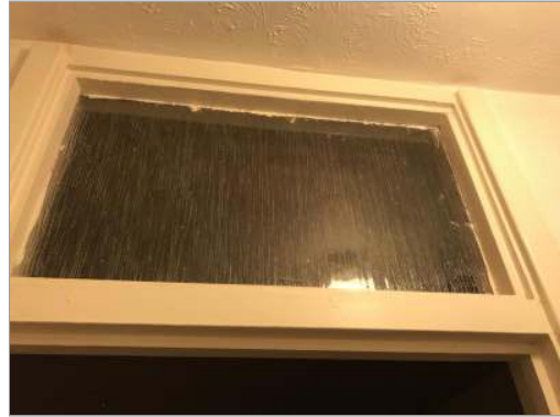
Photo - 99 Ensure internal glazing is made shatterproof.
