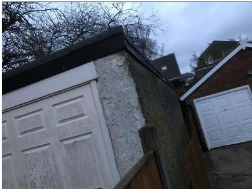
Photo - 126 Blown concrete noted.
