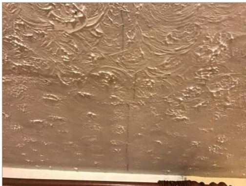
Photo - 68 Joint repairs required to artexed bed 2 ceiling.
