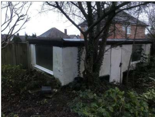
Photo - 116 Blown render noted to walls.
