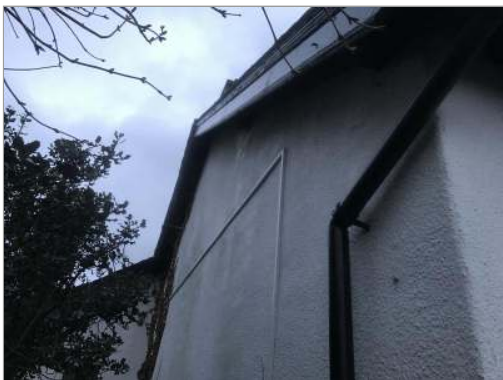
Photo - 22 Patch repairs evident to render.
