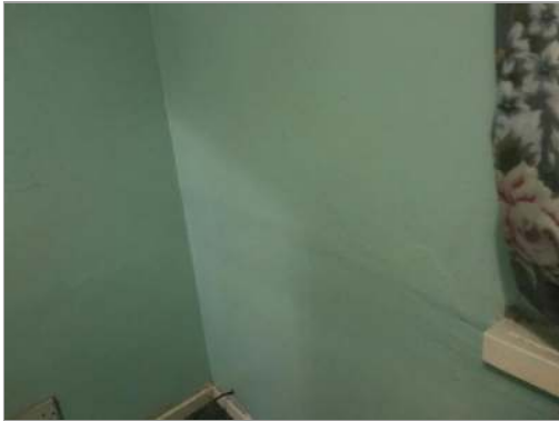
Photo - 79 Historic movement related repairs noted to rear bed 1 window opening area.
