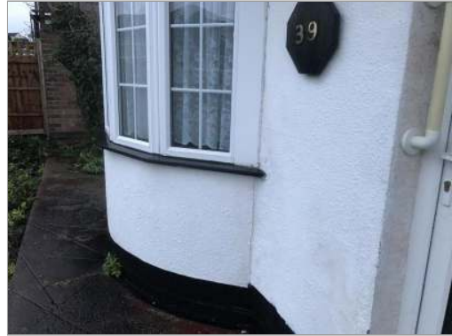
Photo - 19 Low level rising dampness noted to front elevation render.
