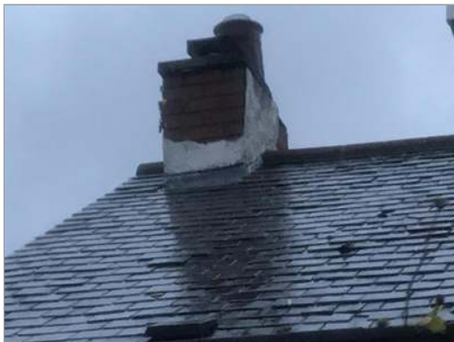
Photo - 1 Blown render noted to stack. Remove.
