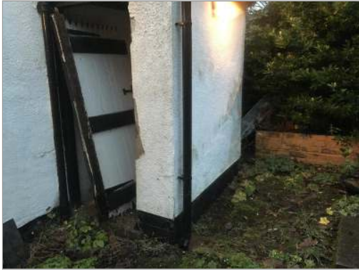
Photo - 26 Penetrative dampness noted to rendered walls.
