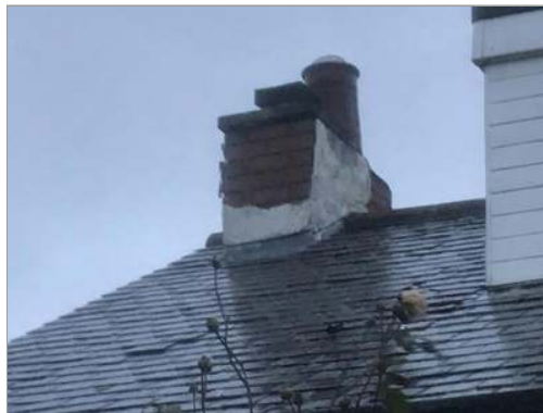
Photo - 2 Leaning stack. Structural monitoring required.
