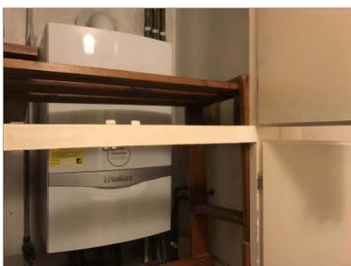
Photo - 114 Modern combi boiler noted to rear airing cupboard adjacent to bathroom.
