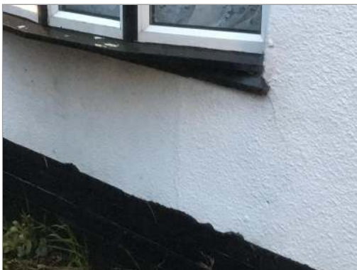
Photo - 30 Moderate movement noted to rear openings.
