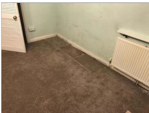
Photo - 85 Pack up sloping floor to low level kitchen.
