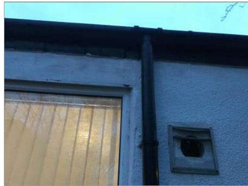
Photo - 29 Leaking gutters noted leading to penetrative dampness around openings.
