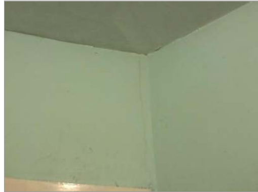
Photo - 80 Movement noted to rear bed 1 wall.
