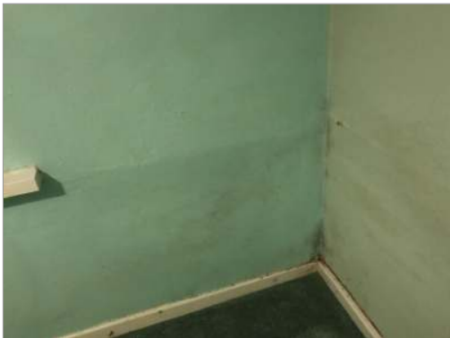
Photo - 81 Low level blown plaster noted to rear bed 1.
