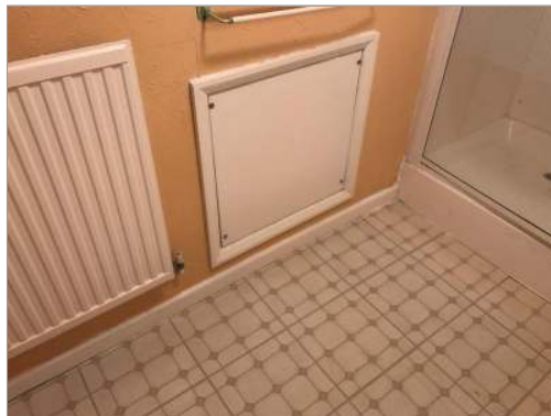
Photo - 60 Eaves hatch to ensuite is screwed shut.
