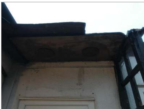
Photo - 33 Renew dilapidated rear door canopy.
