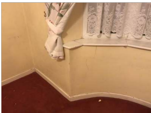
Photo - 75 Moderate movement noted to front lounge bay window wall.
