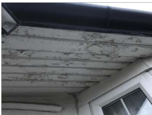
Photo - 39 Penetrative dampness noted to timber soffits from eaves slates and leaking or blocked gutters.
