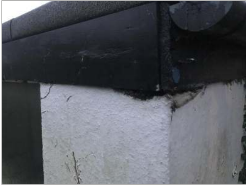
Photo - 120 Splice repairs required to rotten timbers.
