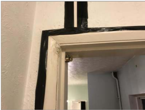
Photo - 100 Movement noted to rear lobby door frame.
