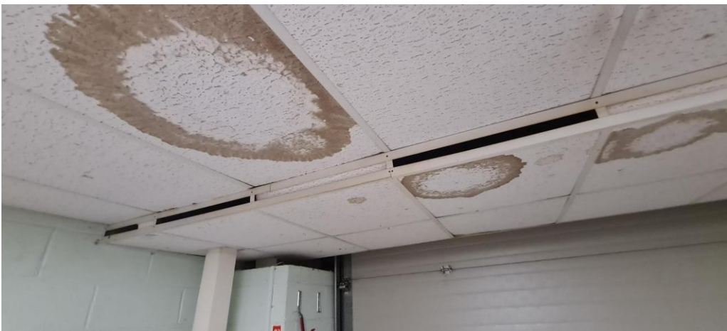
Evidence of past water ingress/leak
