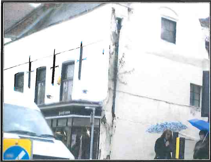
1: Vegetation around downpipe on side elevation.
